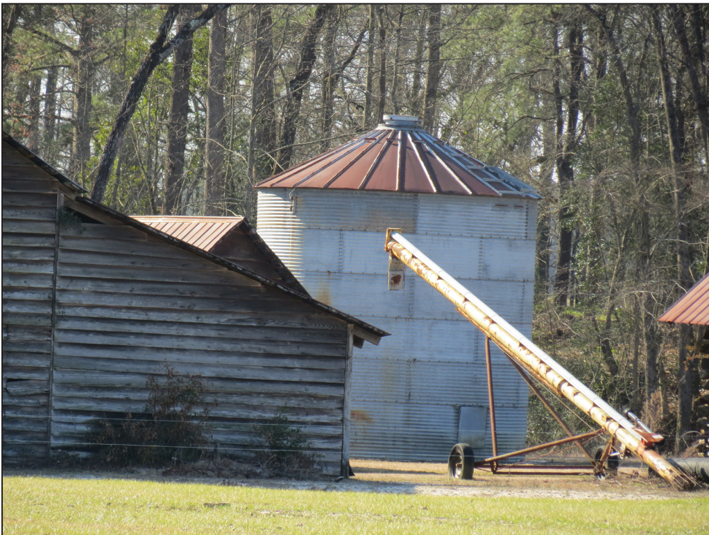
Photograph 4: 20th Century Silo; looking south.
