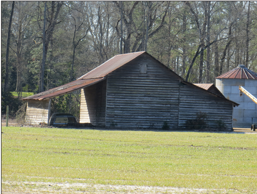
Photograph 1: Northwest and northeast elevation of the 20th Century Barn; looking south.
